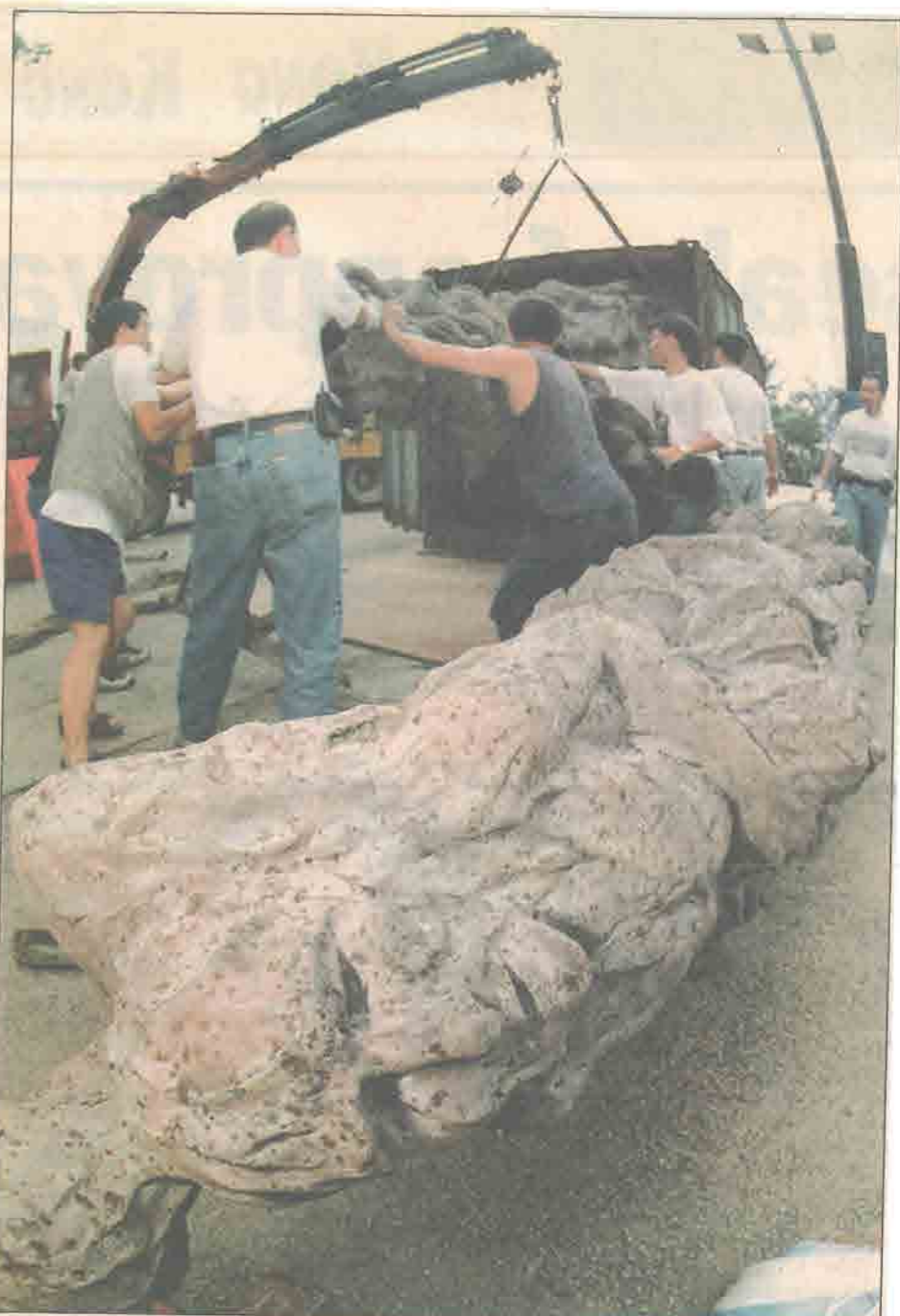
Road to nowhere: Workers dismantle the Pillar of Shame and load it onto a lorry in Victoria Park. It has been stored in a container depot. Its final home is still unknown. PICTURE BY FELIX WONG
