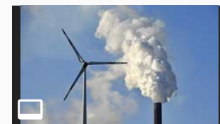
A coal-burning power plant steams behind wind generators in Gelsenkirchen, Germany while the...
